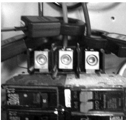
Once the jaws are around the power wire, simply let go of the lever and the sensor “ring” will close around the wire. It’s normal for the sensor to slide down the wire and rest close to the mounting screws.
