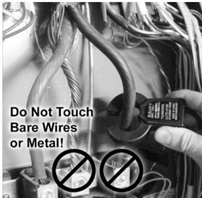
If the electrical service is single phase, you will be installing 2 sensors on the Mains; if it is 3-Phase, use 3 sensors.
