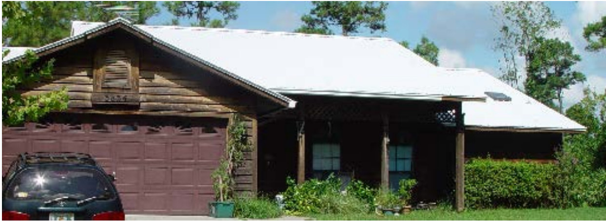
Figure 1. Wood frame retrofit home located in Cocoa, Florida
